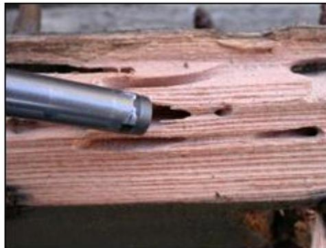
Fig. 6a. Drywood termite damage.
